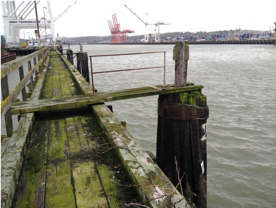
1) South end dolphins (3) and gangway, looking south
