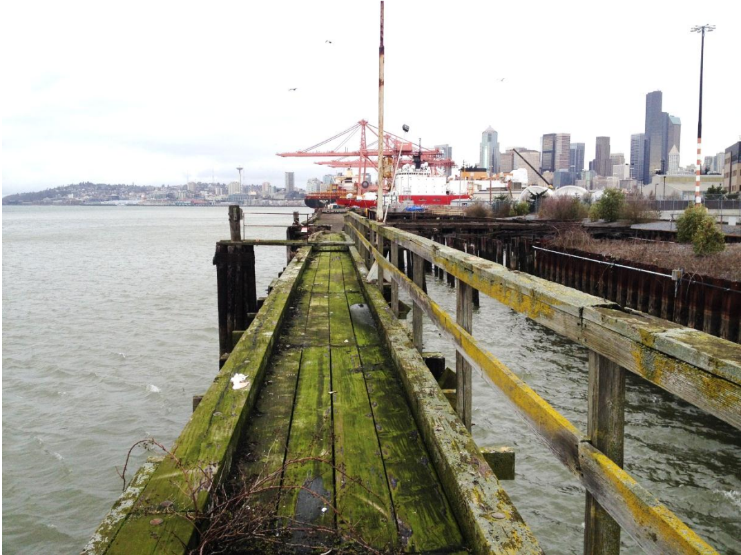
2) South end walkway looking north
